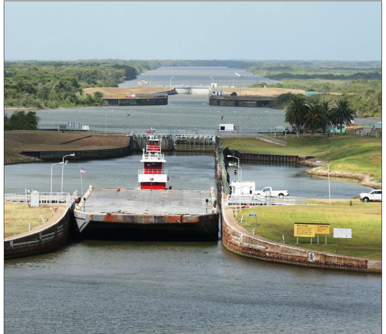
Colorado River Locks, Texas (SWD)
